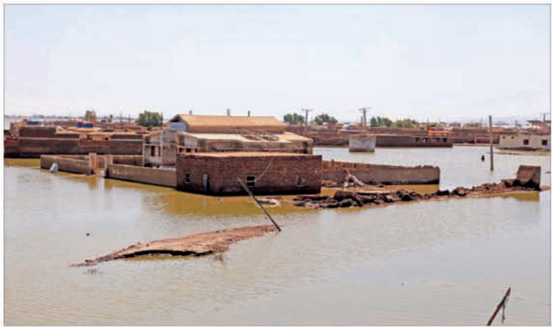
DADU: A melancholy view of unexpected flood disaster where damage houses and mosque submerged in water after deadly flash flood hits the area in Shah Khairpur Nathan (KN) Shah.
