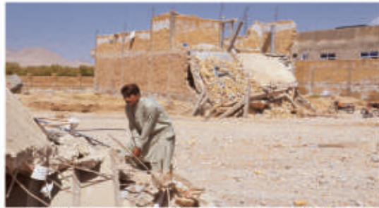
Technical staff engaged in clearing of the highway in Bolan Balochistan: Photo taken from social media
