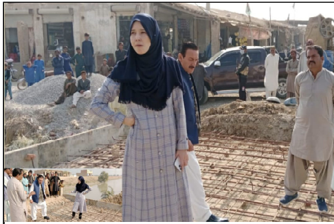
NASERABAD: Deputy Commissioner Batul Asadi is inspecting the under-construction Chhatr.
