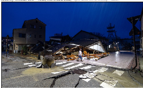
JAPAN: A view of buildings destroyed by the earthquake in Wajima, Ishikawa Prefecture.
