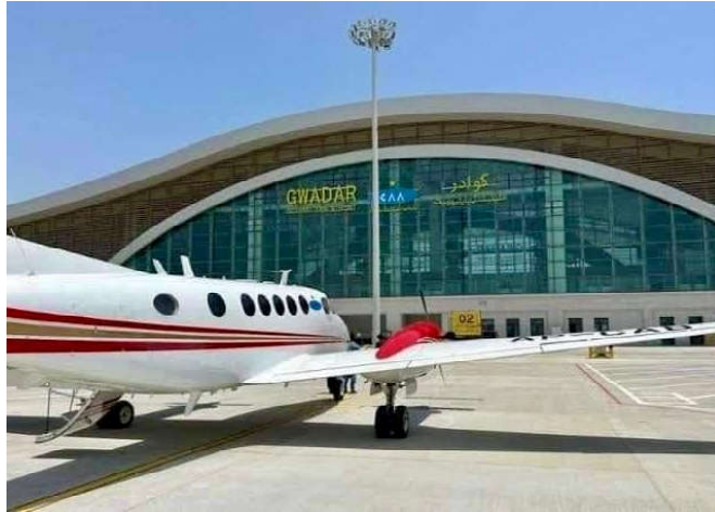
A view of newly constructed Gwadar International Airport (GIA), Photo taken from social media.
