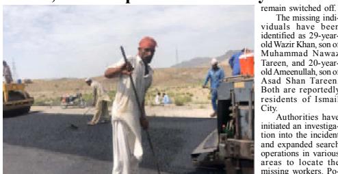
A road construction site with workers and machinery.
