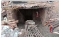
FRONT PAGE Deadly Collapse in Harnai Highlights Perilous Reality...
