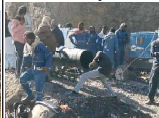
Technical team on the spot for repair of the damaged gas pipeline: Photo Quetta Voice
